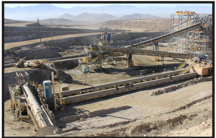
Solids Transfer Systems - Crushing Circuits, Conveyed Products
